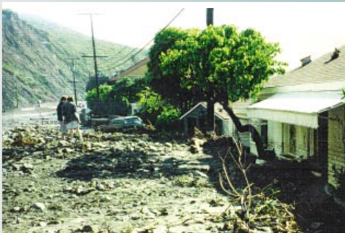
During late May and early June of 1983, a series of debris flows emerged from Rudd Canyon into the community of Farmington, Utah. Although no one was injured, a number of houses were inundated and destroyed by debris flows. Due in part to USGS studies, debris basins were constructed here and elsewhere along the Wasatch Front north of Salt Lake City to prevent subsequent damage. Utah was particularly hard hit by landslides and debris flows during the El Niño events that struck the United States in the early 1980's (Photo: S. Ellen, USGS).
