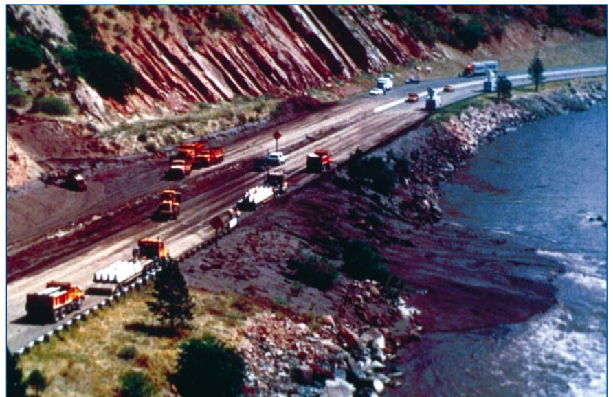
Debris flows like these near Glenwood Springs, Colorado, are a consequence of heavy rainfall on burned hillsides. In addition to personal injuries and damage to 30 vehicles engulfed by these flows, transportation along the Interstate 70 corridor was brought to a standstill for a day, and business and emergency operations in the Glenwood Springs area were seriously impeded (Photo: Jim Scheidt, U.S. Bureau of Land Management).
